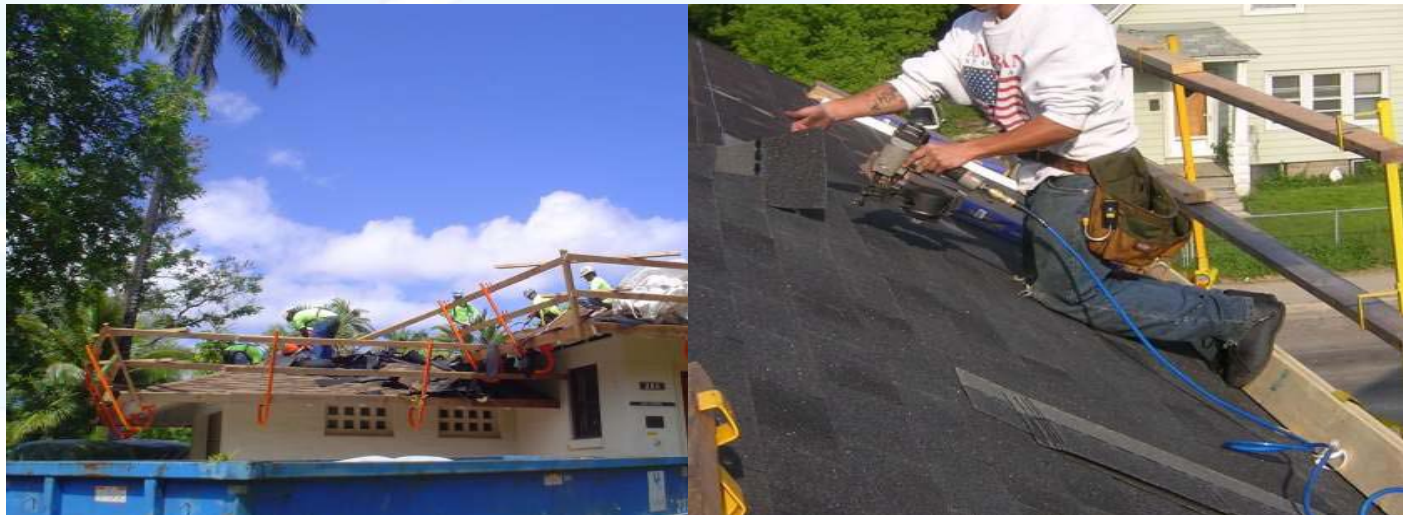
Guardrails in place during re-roofing activities.
