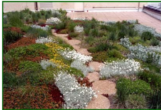
Chicago's City Hall Bennett & Brosseau Roofing
