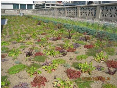
Chicago Cultural Center, Anderson & Shah Roofing
