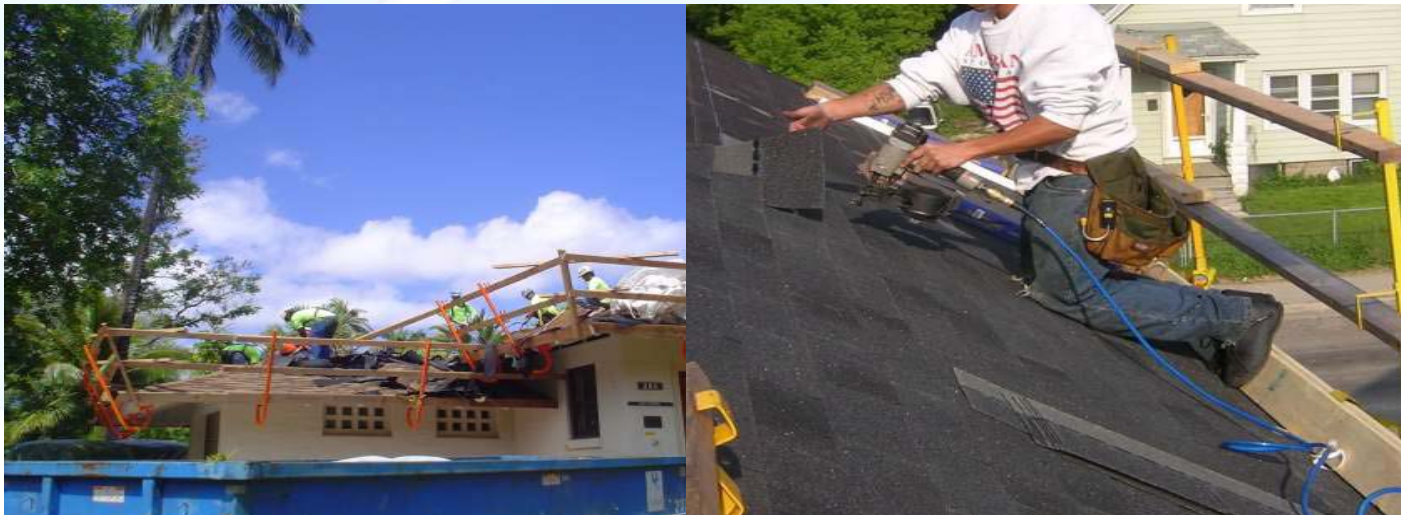
Guardrails in place during re-roofing activities.
