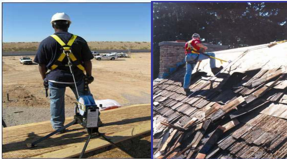
PFAS in use during roofing and re-roofing activities.
