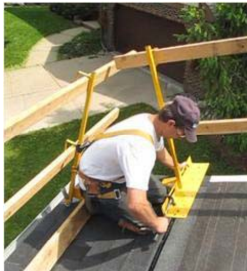
5) Secure Positioning Nail
