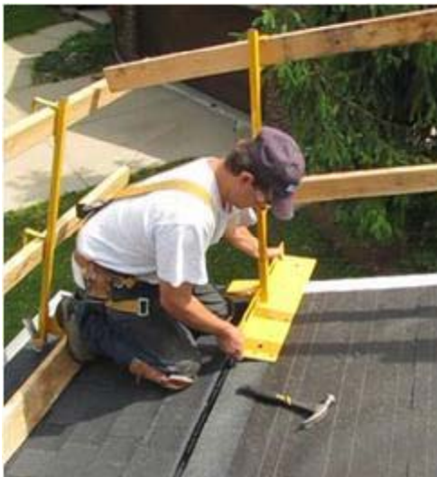
4) Move Bracket Down to Positioning Nail
