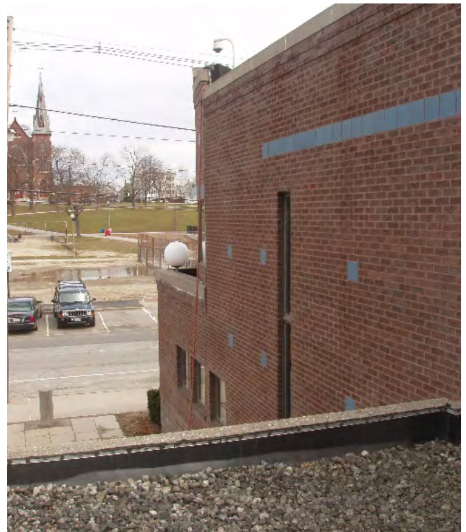
Photograph 3—Membrane Shrinkage: Notice the roofing membrane being pulled away from the cant strip.
