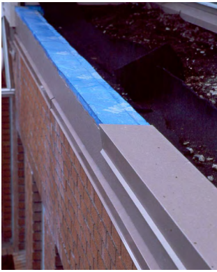
Photograph 1—Excellent Water Management: Notice the membrane under the coping. Notice the slope to the interior. And, notice the drip edges.
