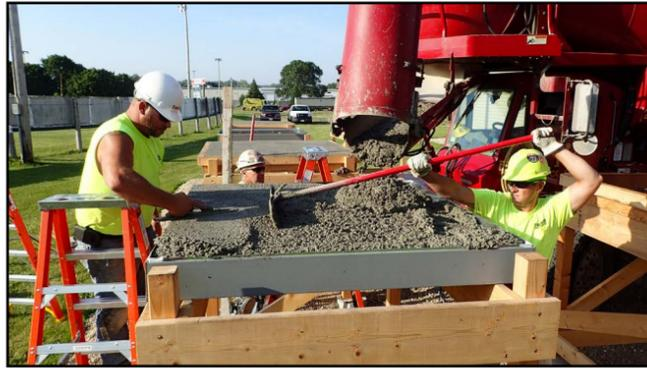
Photo 1. A large general contractor was utilized to provide concrete slab assembly, placement and finishing. These slabs are the exterior slabs, exposed to the full weather at SRI Consultants facility Wisconsin. SRI Photo
