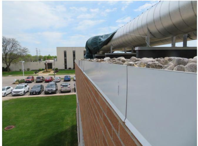
*Photo 1: Edge metal must be higher than ballast (2-inch minimum).
