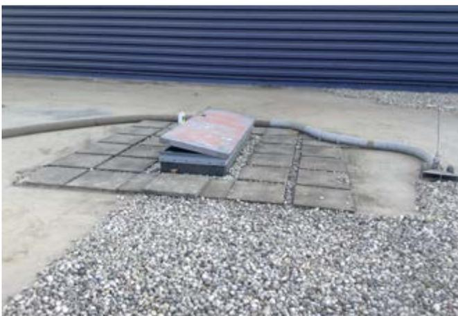
Example of access to roof via a hatch. When not in use, should be maintained in the closed position. (Photo courtesy of Safety Check, Inc.)
